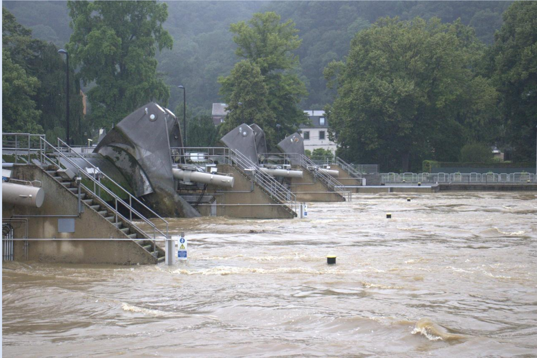
Photo 1. The locks are wide open, the water rises in Belgium on July 15th 2021
