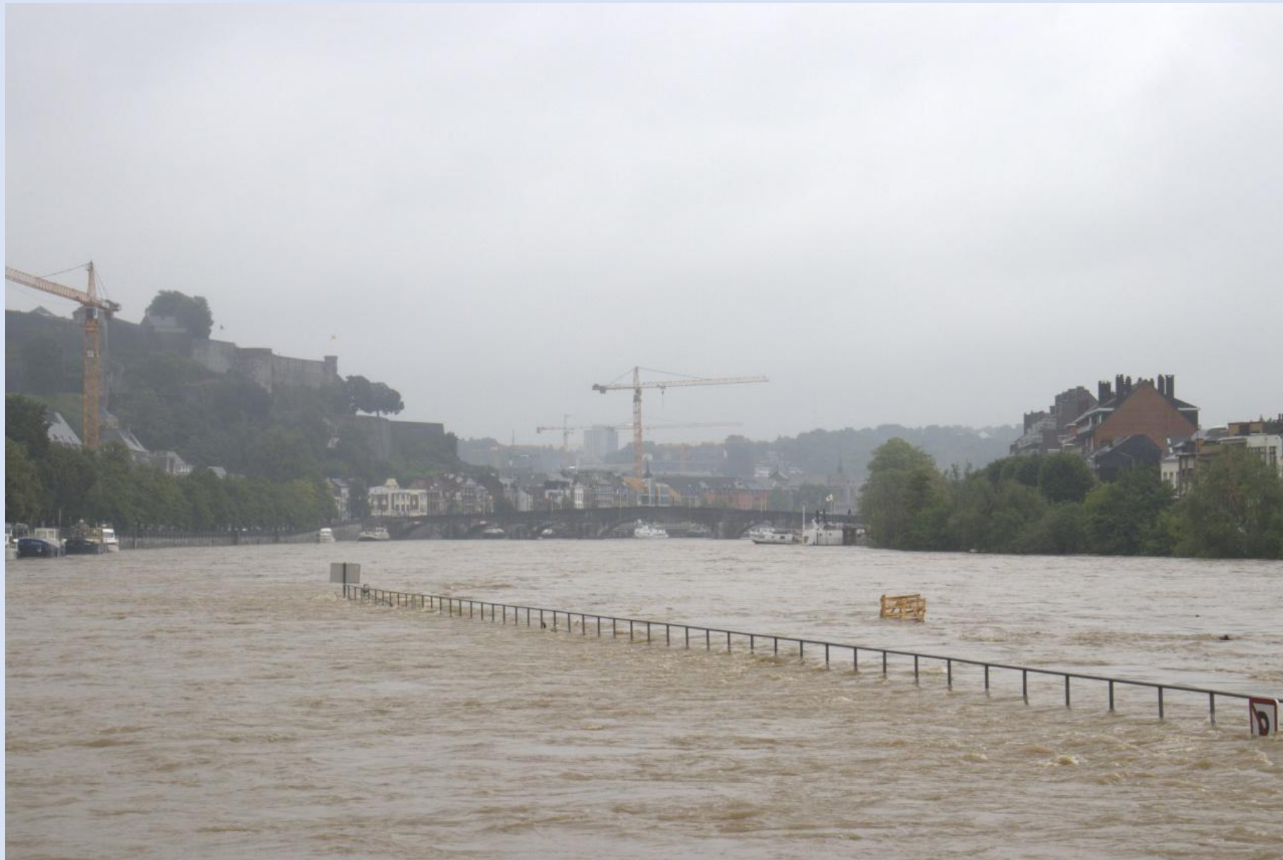
Photo 2. The Meuse enters Namur and takes with it the debris from the houses
